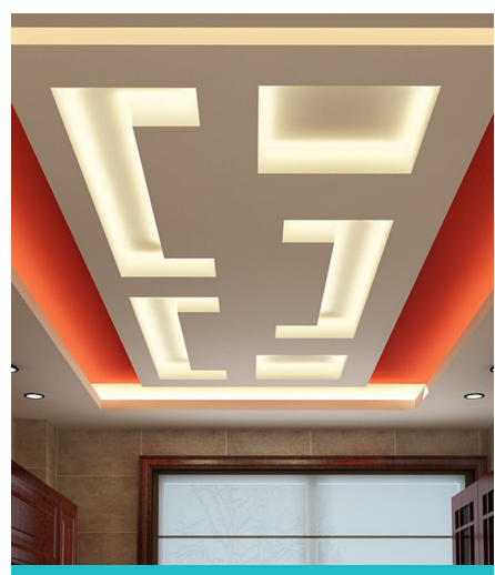
FALSE CEILING & GYPSUM WORK
