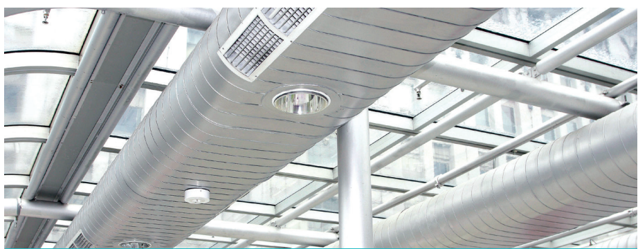
AC DUCT INSTALLATION
